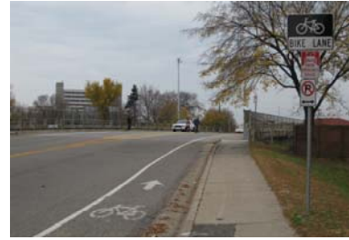
Above: Bike lane along 20 th Avenue South.
