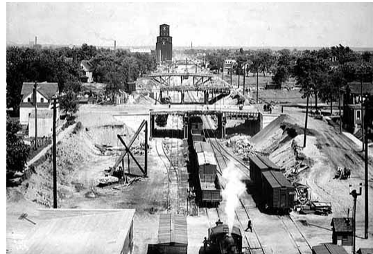
Above: Bridge construction at Portland Avenue (1915).
