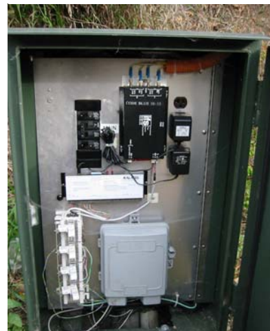
Above: A fiber optic cabinet along the Midtown Greenway
