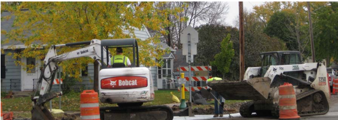
Above: Construction equipment along the RiverLake Greenway.
