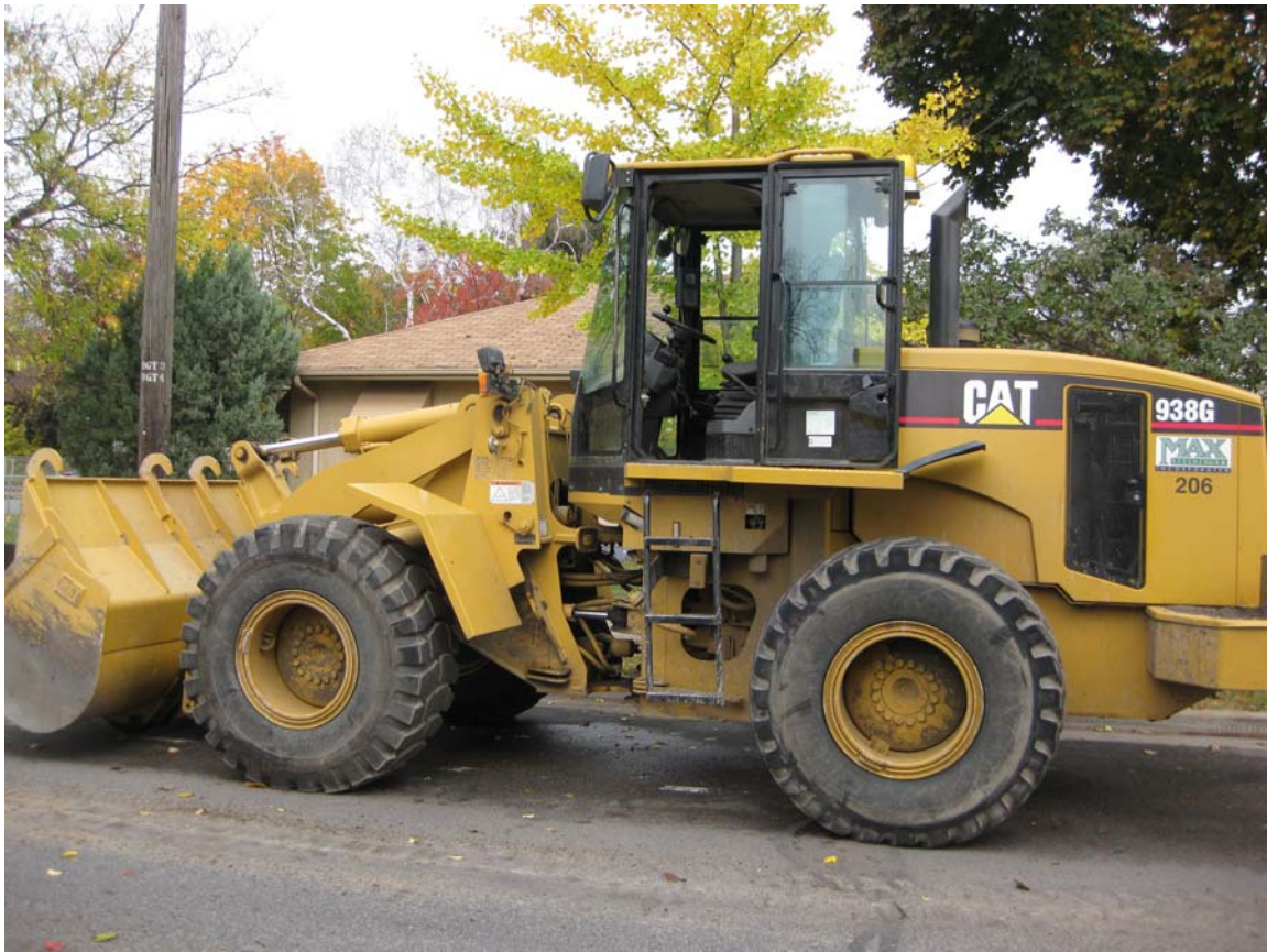
Above: Construction equipment along the RiverLake Greenway.
