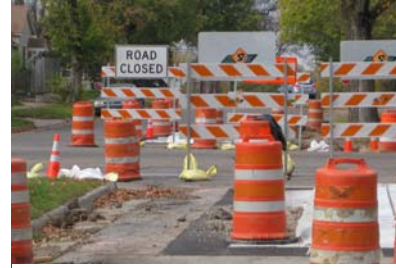
Above: Road closure signs along a new bike route.
