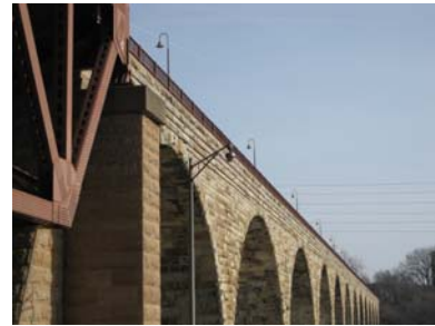
Above: Stone Arch Bridge
