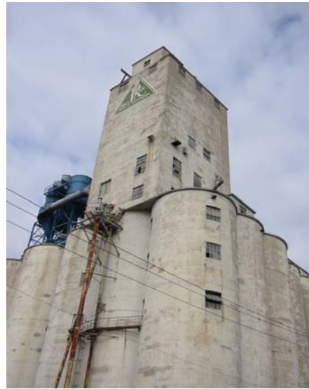
Above: CEPRO grain elevator before it was demolished. The county purchase of the grain elevator eliminated the need for rail service and allowed for Phase 2 of the trail to be constructed.
