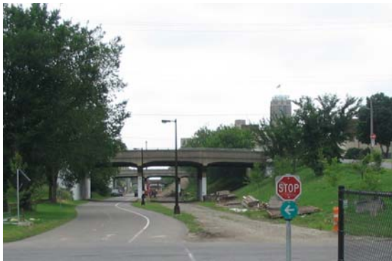
Above: Midtown Greenway bridges today.
