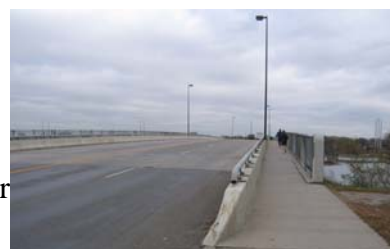
Above: The Plymouth Avenue Bridge will have bike lanes installed in 2011.
