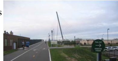
Above: Midtown Greenway Bridge Over Hiawatha.
