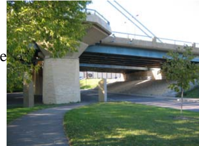
Above: Hennepin Avenue Bridge
