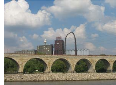
Above: Stone Arch Bridge
