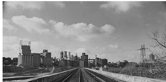
Above: The bridge had two sets of tracks and served passenger trains until 1978. 1965 photo courtesy of the Minnesota Historical Society. Photo by Alan Ominski.
