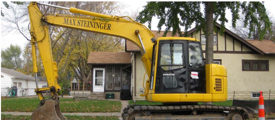
Above: Construction equipment along the RiverLake Greenway.
