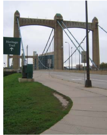
Photo: The Hennepin Avenue Bridge today.
