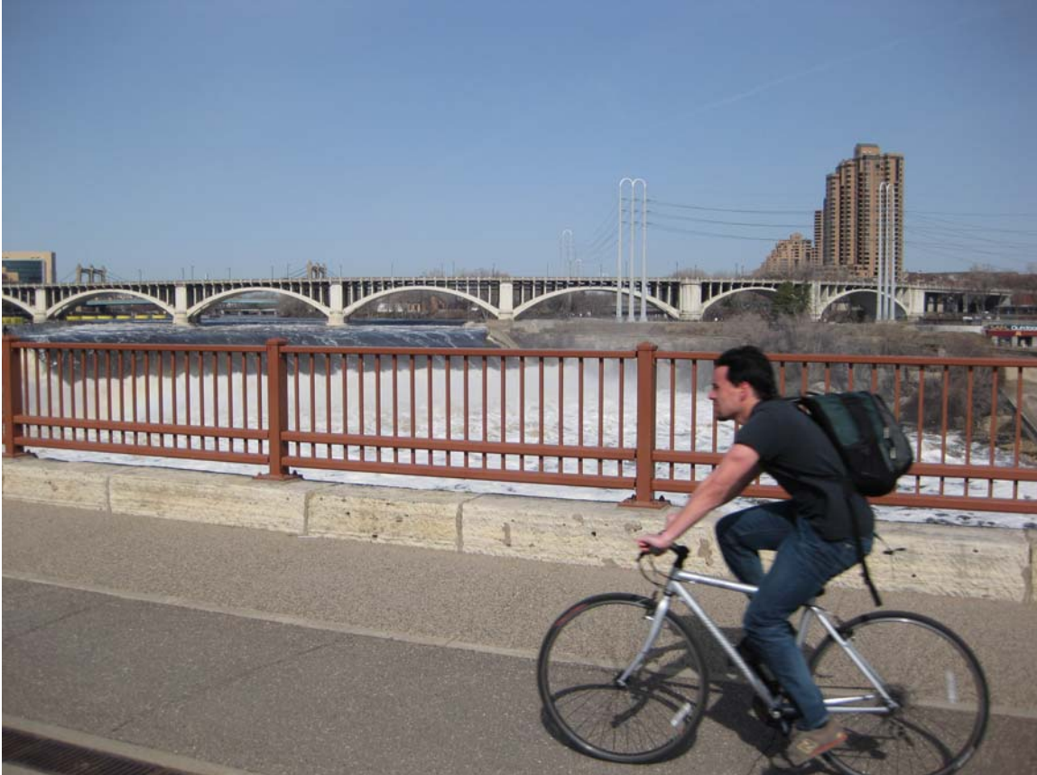
Above: Stone Arch Bridge
