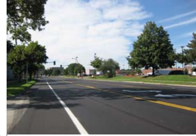
Above: Bicycle lanes on 26 th Avenue South.
