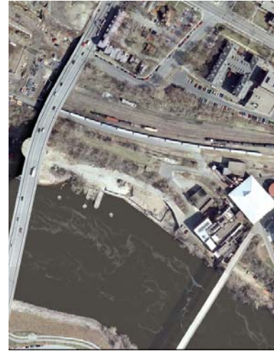
Above: 10 th Ave Bridge and Bridge #9 today.
