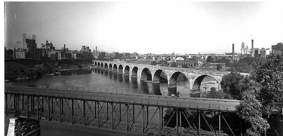
Above: 1918 Photo showing original 10th Avenue Bridge, Stone Arch Bridge and new 3rd Avenue Bridge. Photo courtesy of the Minnesota Historical Society.
