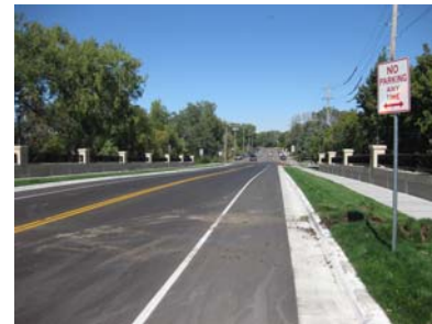
Above: Marshall Street NE Bridge with striped shoulder
